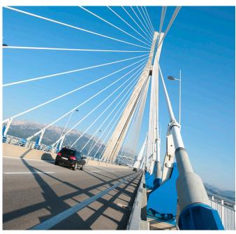
The Rion-Antirion Bridge in Greece is one of more than 20 bridges where we supplied Stay Cable Dampers
